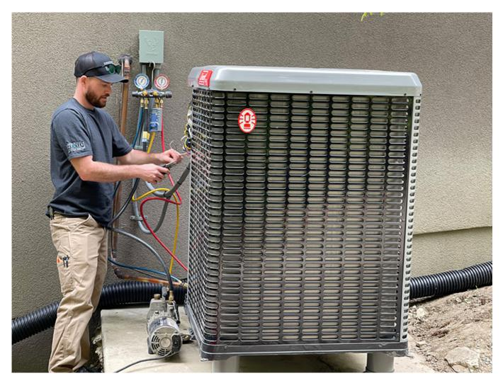
Like air conditioners running in reverse, heat pumps such as the one being installed here use refrigerants to capture heat from the outdoors and move it indoors to heat the house.
