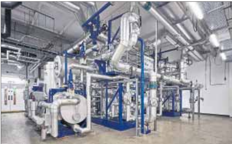
Below: Star Refrigeration's heat pump at the heart of the West Dunbartonshire Energy Centre
