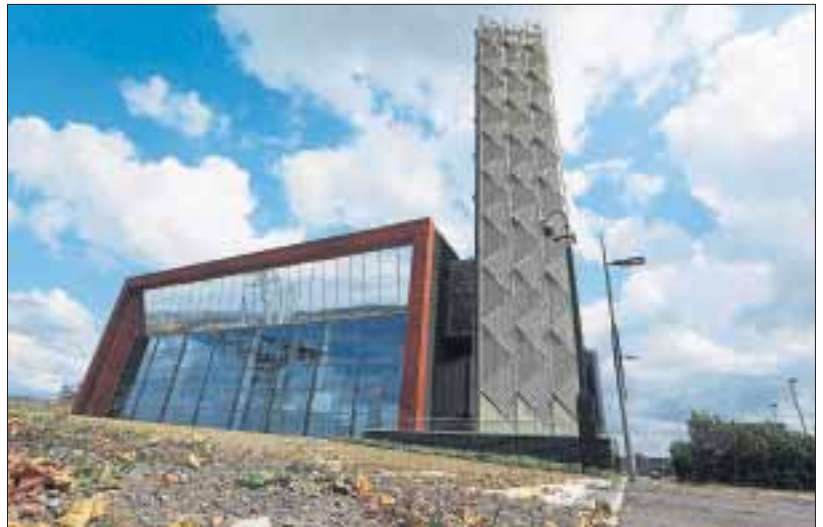
The district heating system at Queens Quay, pictured above, now officially known as the West Dunbartonshire Energy Centre, is home to the UK's largest water source heat pump, providing affordable low carbon heating and hot water to around 1200 homes and businesses via a network created by Vital Energy. Right: Work continues on housing at Queens Quay
