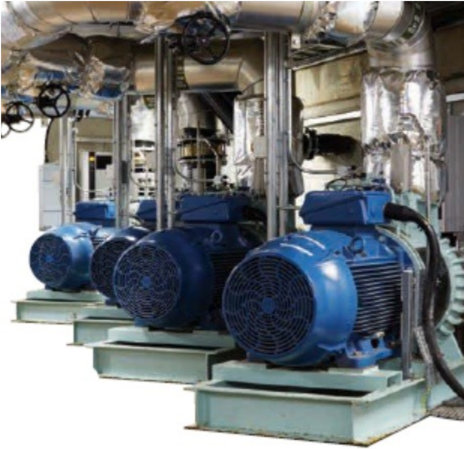
The abstraction pumps drawing water from the River Clyde. (Image: Vital Energi) »
