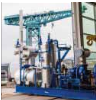
Star Refrigeration's pump system being installed at Queens Quay
